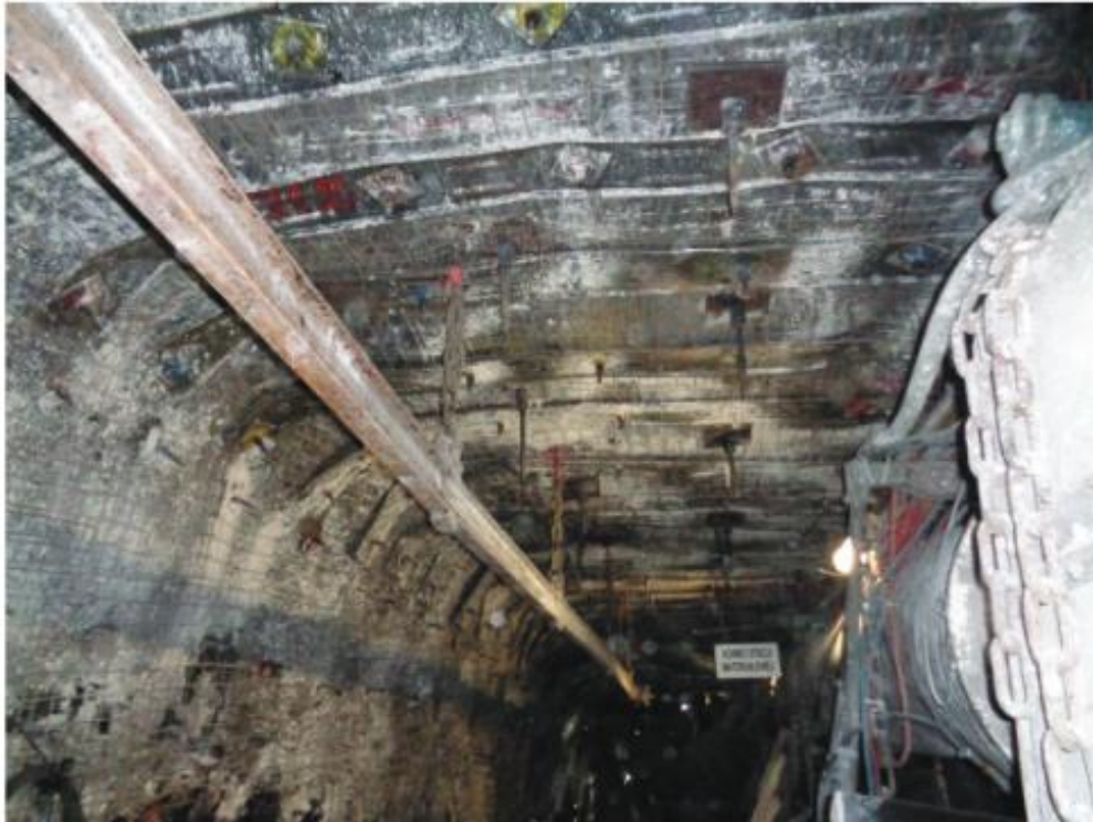
Fig. 3. Rock and cable bolts with mesh installed in the exploratory roadway at LW Bogdanka S.A. (photo by M. Antoniuk) from (Rak Z and Stascia 2020).
