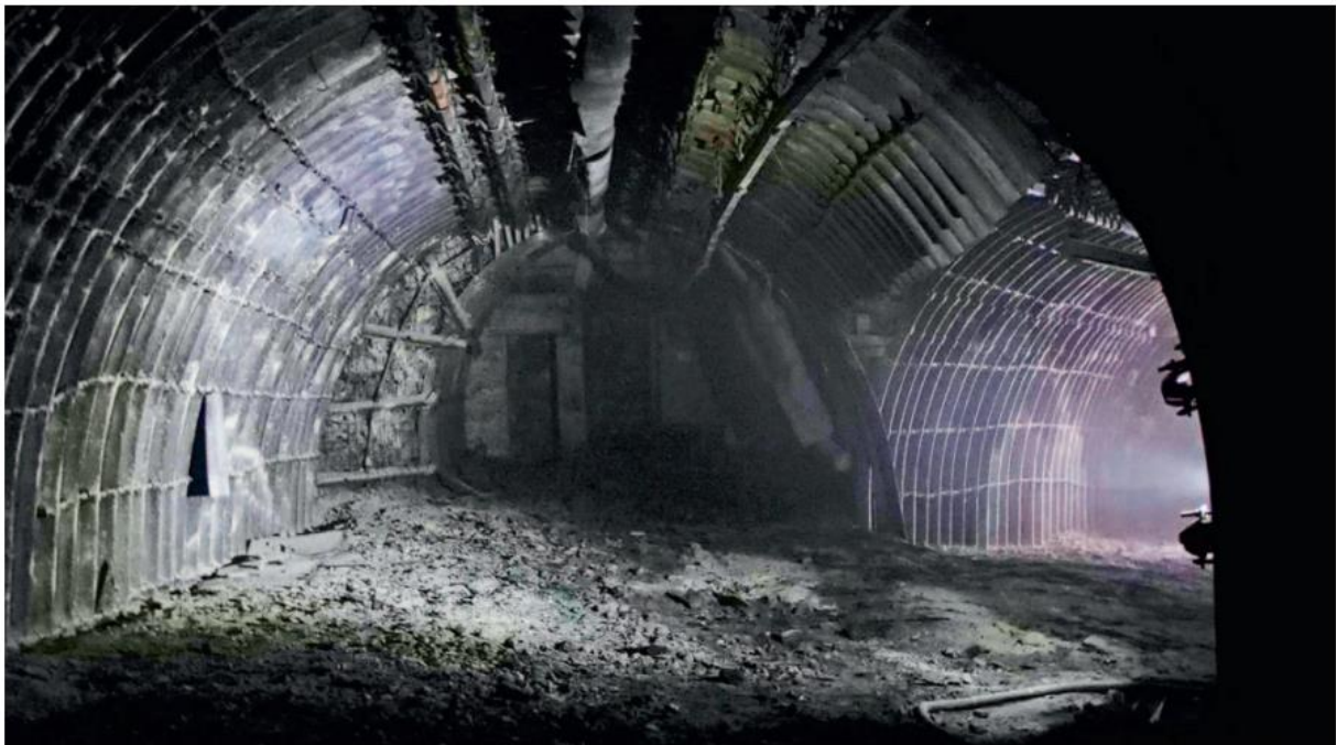
Fig. 2. View of an example intersection of horizontal excavations protected by a typical steel arch support. (Inżynieria Górnicza 2020/1).
