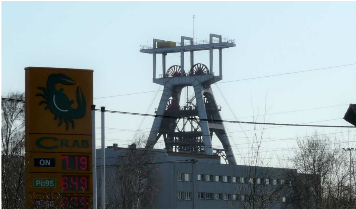
Fig. 61 KWK "Budryk" – headframe of Shaft III [14]
