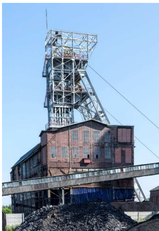
Fig. 36 ZG "Eko-Plus" - strut tower of the "Kopernik" shaft on the premises of the main plant, 2013 [12]
