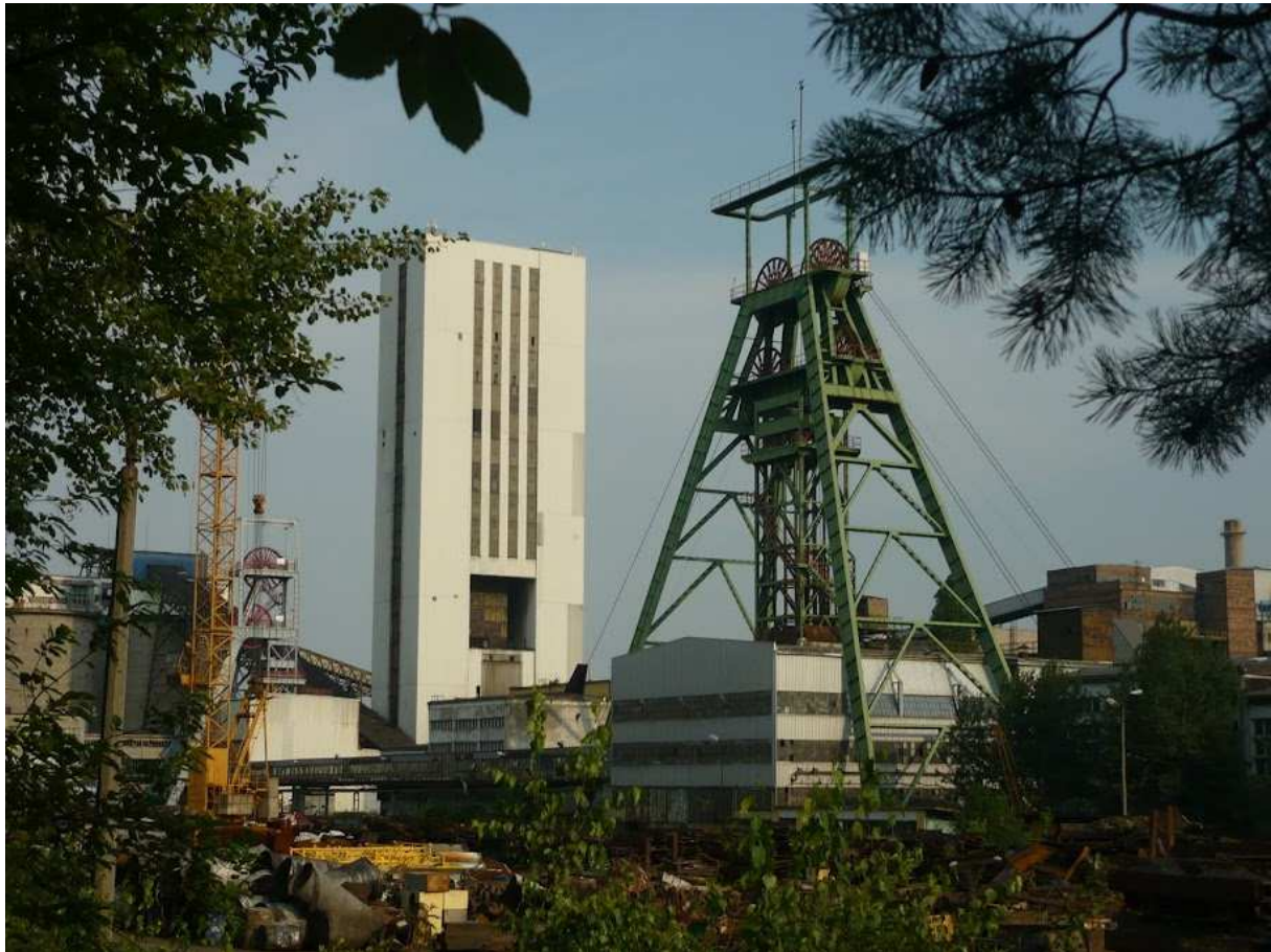
Fig. 67 "Halemba" Section – Tower headframe of Shaft "Grunwald III", state in 2012 [14]
