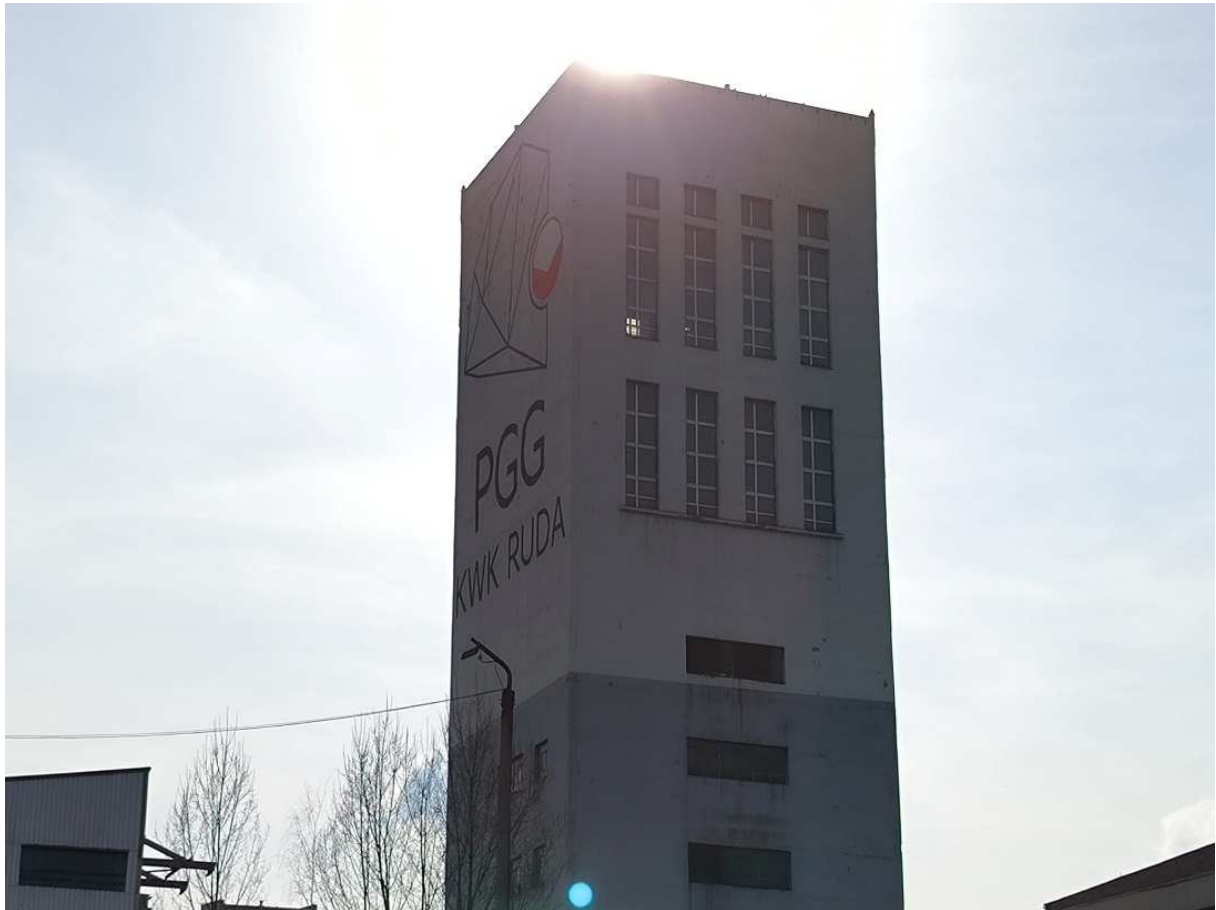
Fig. 24 Ruch Bielszowice division - Shaft III tower, as of 2023 [14]
