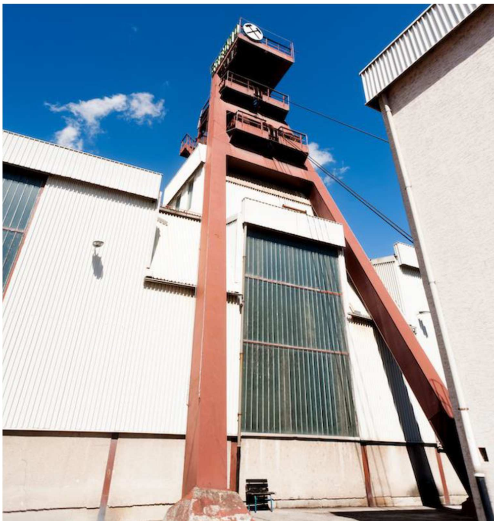
Fig. 55 Transport Shaft Nove Preloge - NOP
