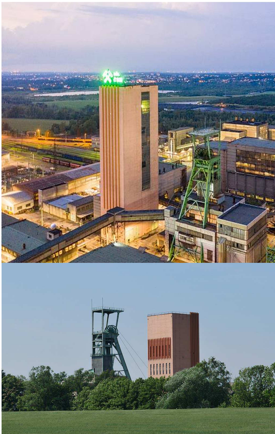
Fig. 46 Shafts of the Sever and Jih mining plants
