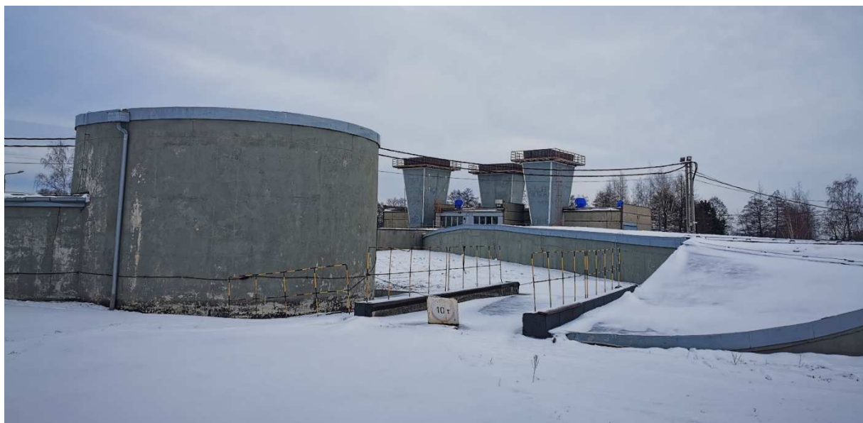
Fig. 22 Pniówek Coal Mine - Shaft V, Channel S and main fan station with diffusers [1]
