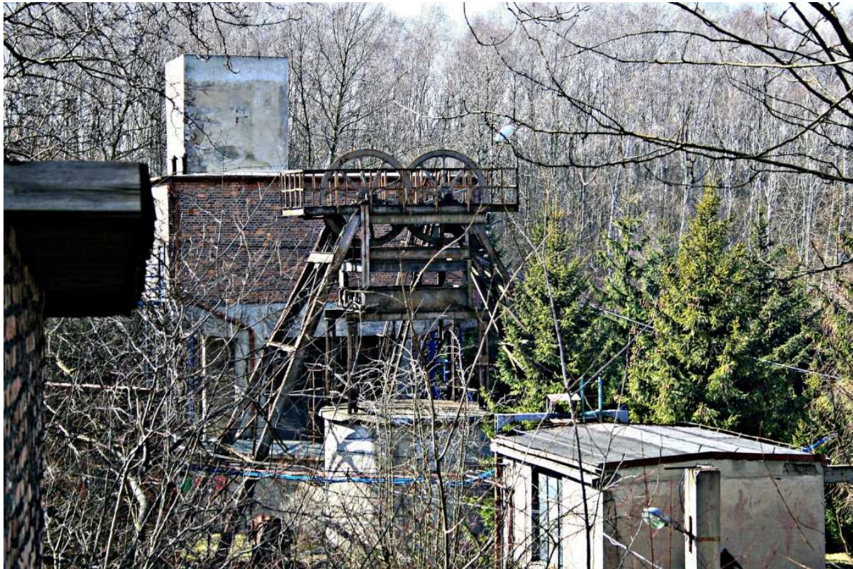
Fig. 34 ZG "Siltech" - peripheral shaft "Mikołaj" and the main fan station in Rokitnica, 2018 [15]
