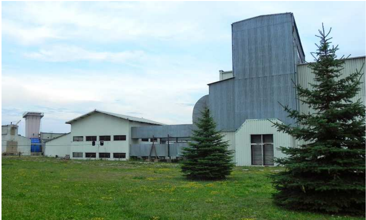
Fig. 43 LW "Bogdanka" building above the shaft of Shaft 1.5 in the "Nadrybie" Division, 2014 [12]
