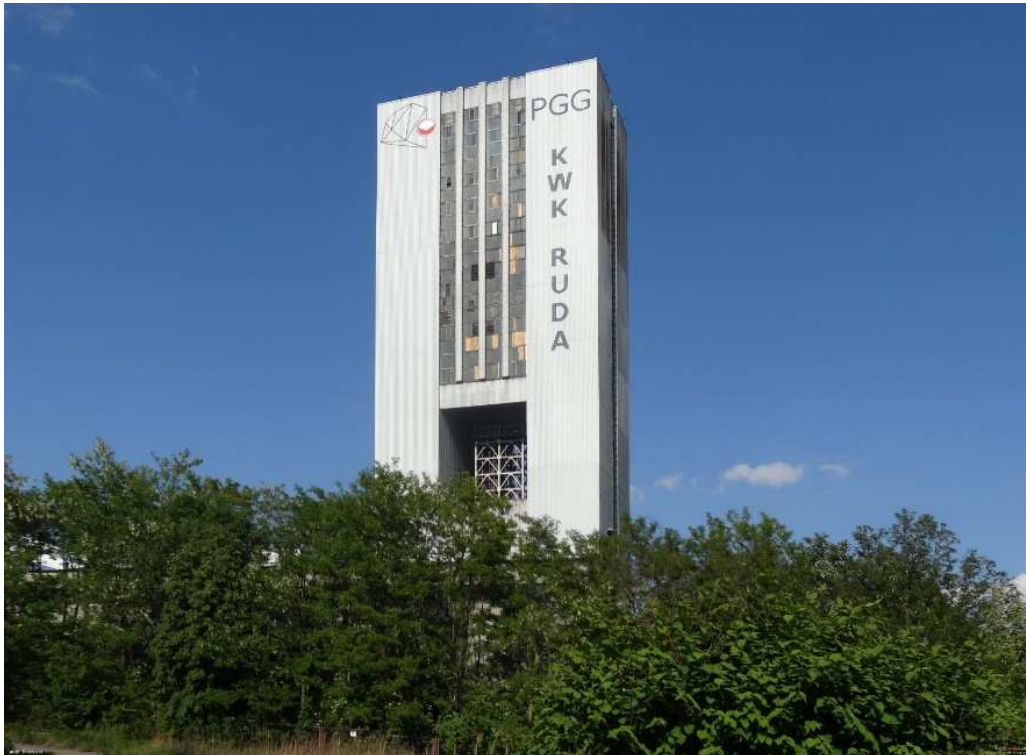
Fig. 69 "Bielszowice" Section – Headframe of Shaft V, state in 2024 [20]
