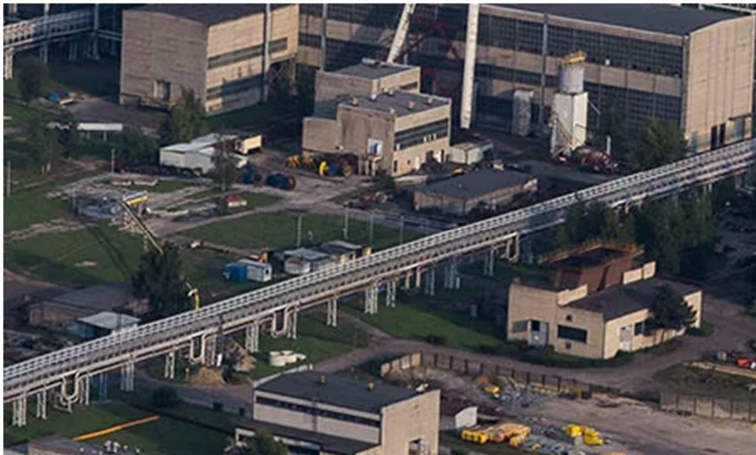
Fig. 59 KWK "Budryk" – top of Shaft II and main fan station, 2020 [3]
