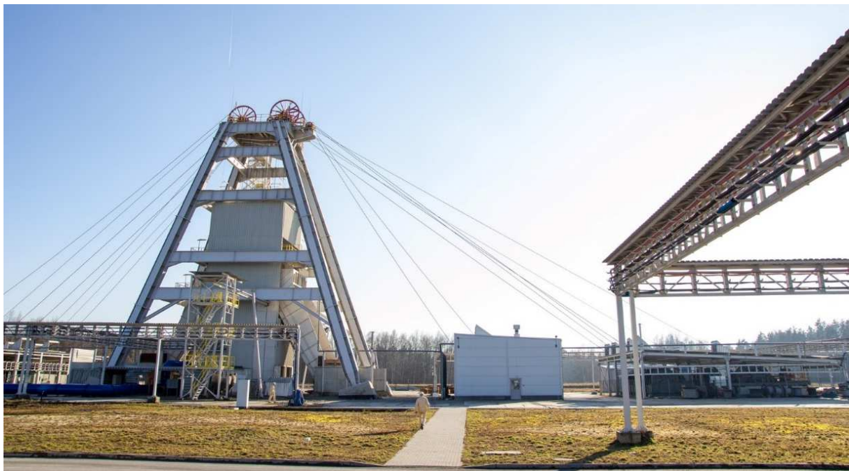
Fig. 28 ZG Sobieski mining plant - trestle tower of the deepened peripheral shaft "Grzegorz", 2024 [6]
