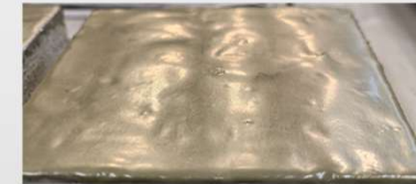
C20/25 + Sikagard M790 after water erosion
