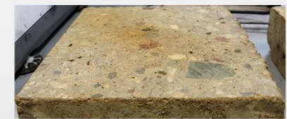
C20/25 after mine water erosion
