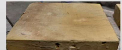
C20/25 + Sikagard WallCoat T after mine water erosion
