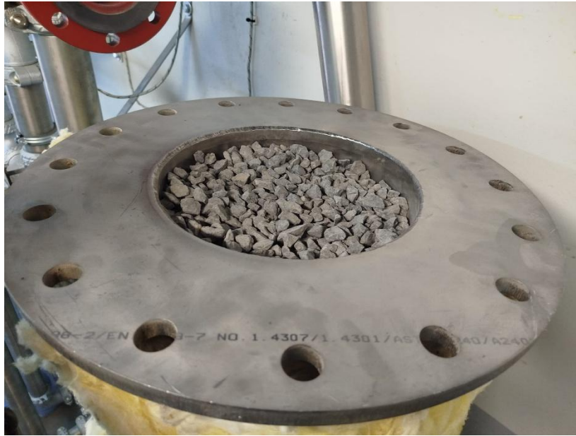
Figure 4 Thermal storage bed.
