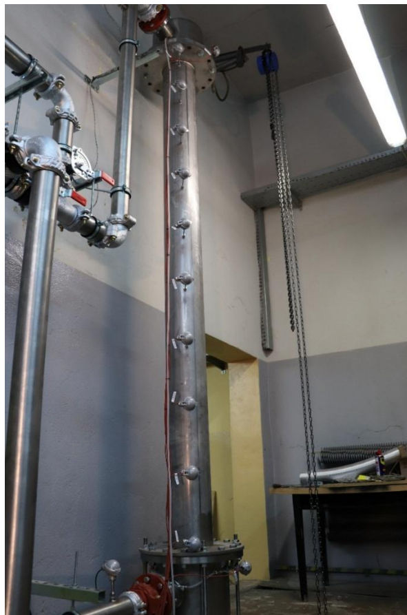
Figure 1 Thermal Energy Storage tank with a Porous Bed at Silesian University of Technology.
