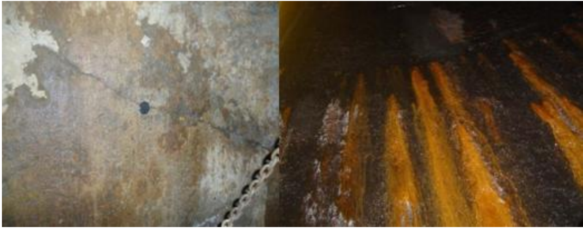
Figure 1 Degraded shaft lining after several decades of operation[17]
